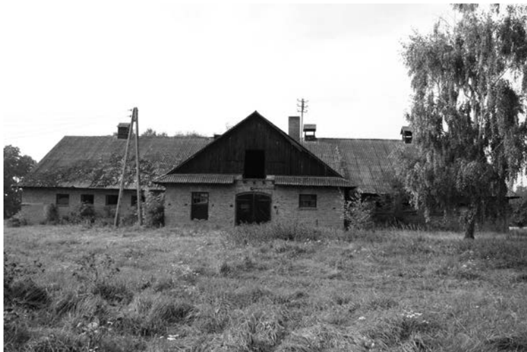
FIGURE 4. A derelict sheepfold on the former manor estate – a characteristic element of the historical landscape of Rogalin. There is a proposal to convert this building into a tourist facility (photo by M. Jaroszevska)
