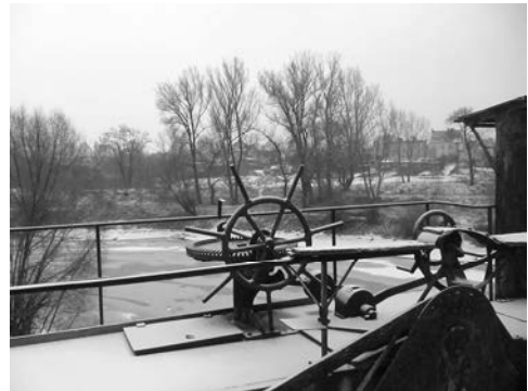
FIGURE 3. Fragment of the port construction in Malczyce (photo by I. Niedźwiecka-Filipiak, 2007)
