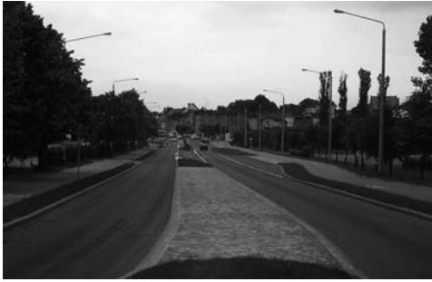
FIGURE 4. An example of a comprehensive set of traffic-calming measures installed along national road 20 in Kościerzyna, Poland (J. Żukowska)
